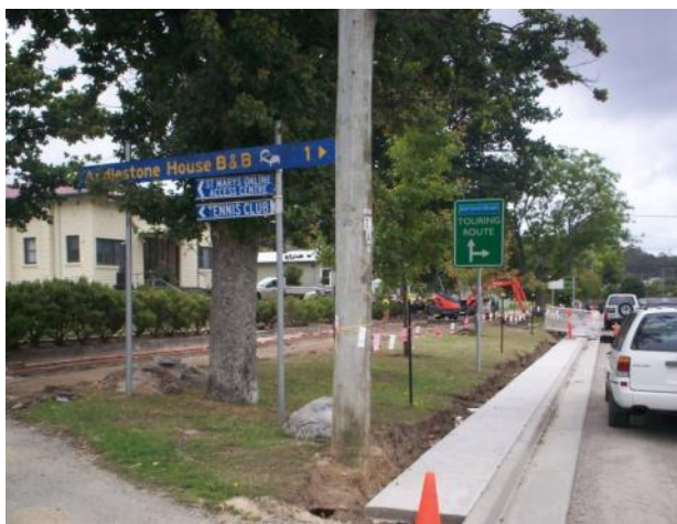
Main Street makeover in progress.
