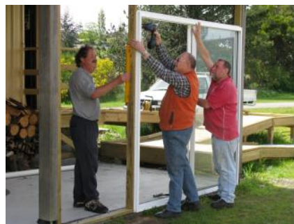
Work on the annex is progressing well.
