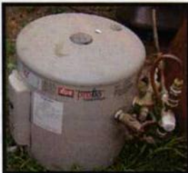
Small hot water cylinder
