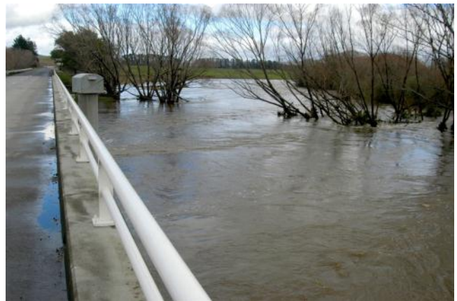
Break O'Day River bridge at Killymoon.
