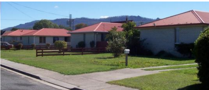
Housing Commission units. Groom St. St Marys.
