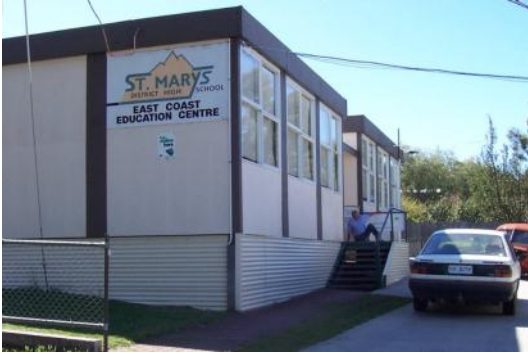
St Marys On-line Access Centre.
