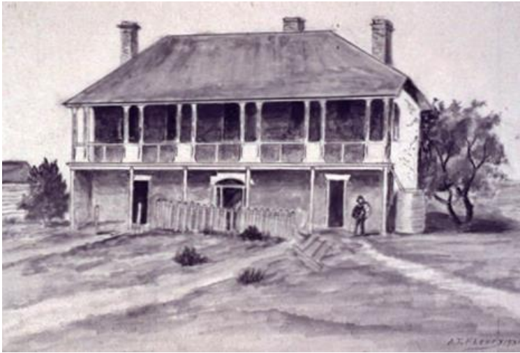
Said to be haunted, Addington Lodge, New Norfolk. (W.L. Crowther Library, SLT)
