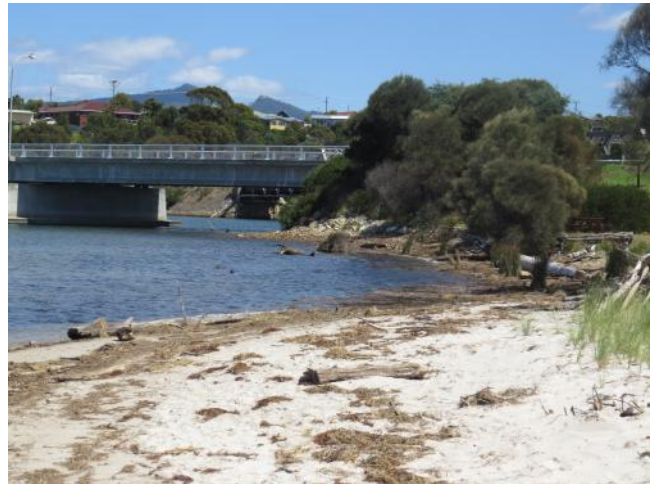
Erosion adjacent to new bridge
